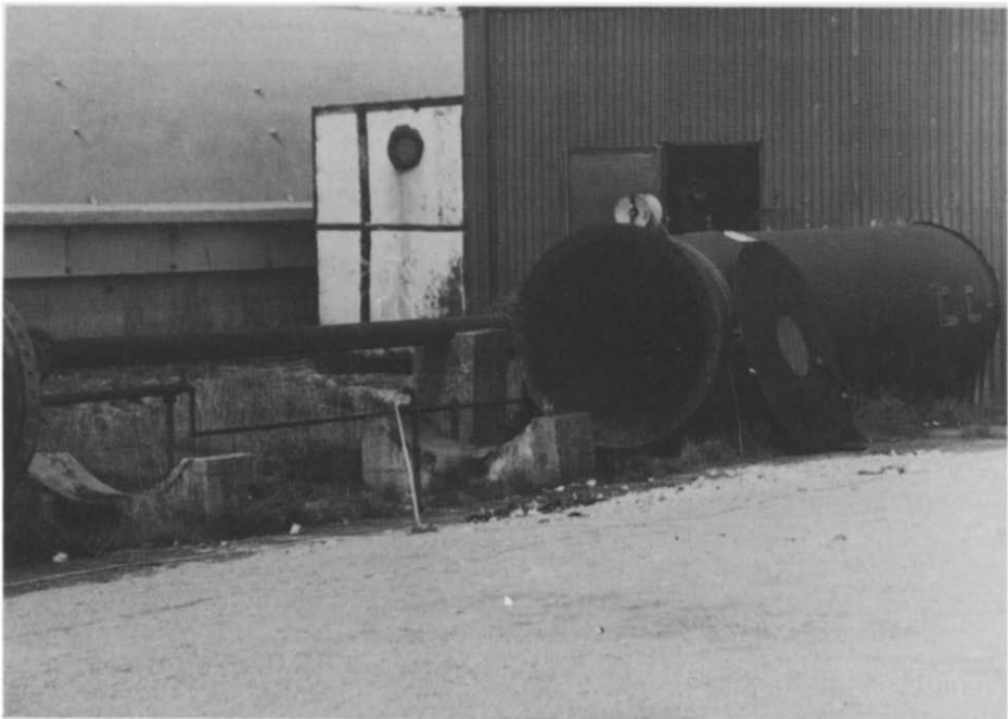
Fig. 4. The 1.2-m diameter steel gallery.
